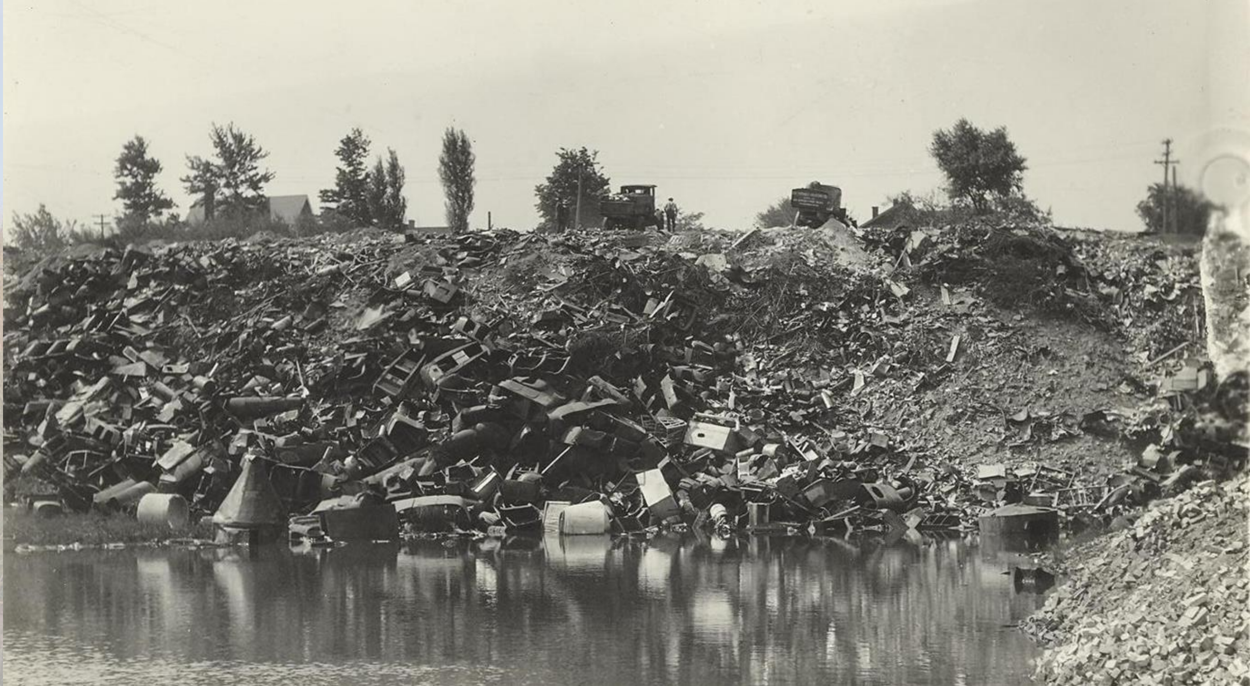
Source: City of Grand Rapids Community Archives and Research Center
