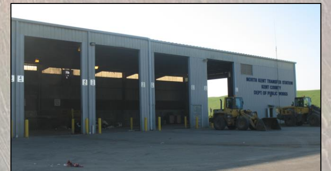
North Kent Transfer Station
