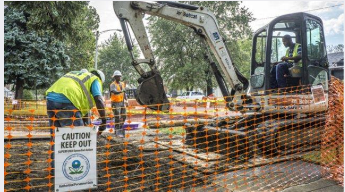
Removal of lead and arsenic contaminated soil from the USS Lead Site in East Chicago, IN (EPA, 2025)
