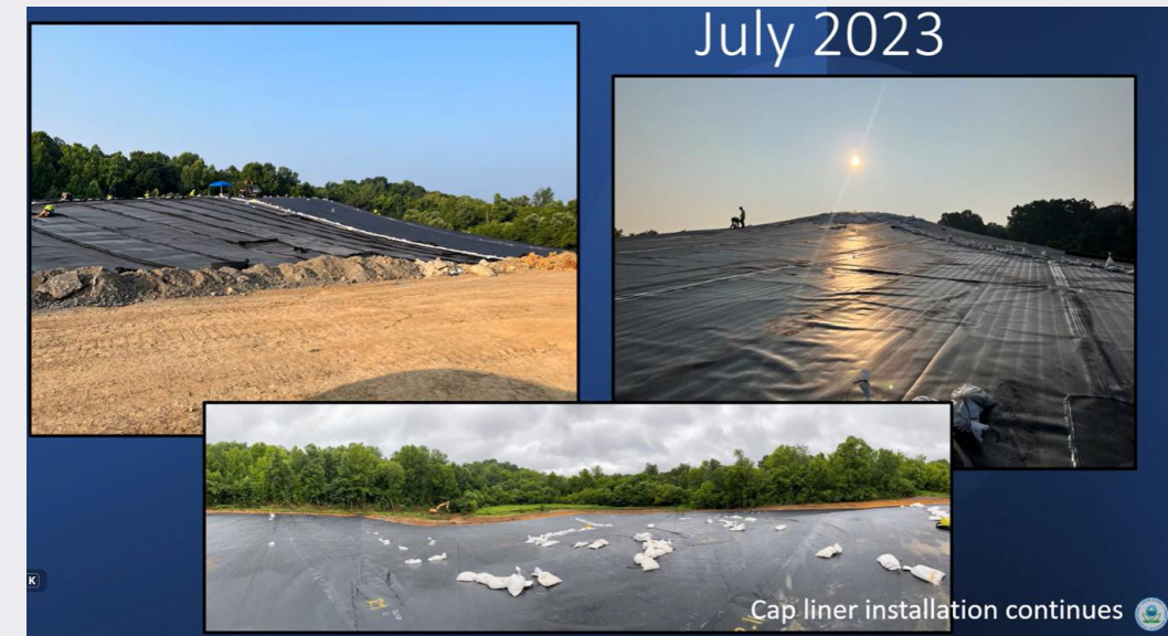
Cap Liner Installation at Smokey Mountain Smelters Superfund Site (EPA, 2023)
