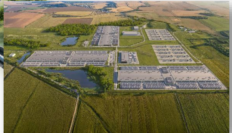
Related Digital, Oracle Data Center in Saline Township
