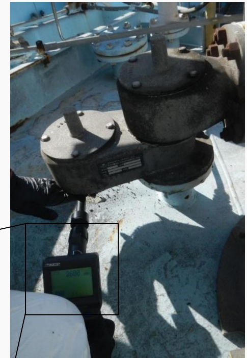
Inspectors using an FID observed detectable emissions (>500 ppm) from relief device on a fixed-roof tank
